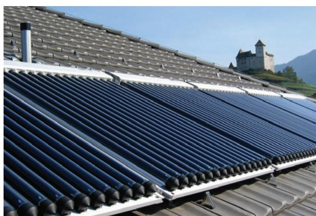
OPC naturally has a mounting system for flat roofs as well, and also for Eternit and wall mounting. For a flat roof, the OPC collector be-
